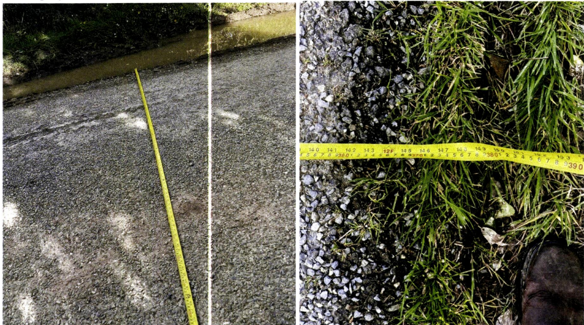
Photographs of L-6175-0 local public road width
